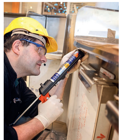
Fig. 9 Application of Sikaflex®-291i
